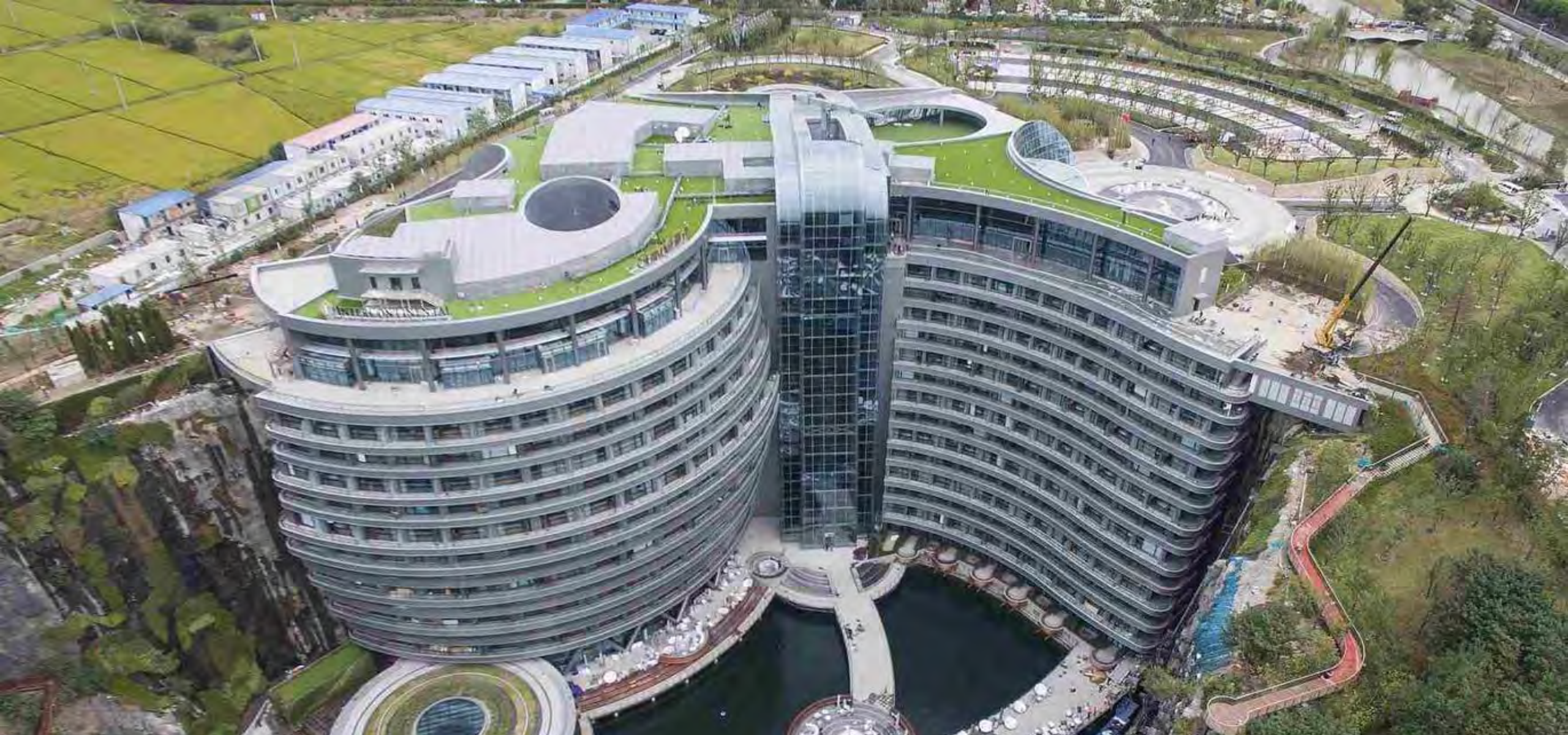
Quarry Hotel: InterContinental Shanghai Wonderland Songjiang, Shanghai, China
